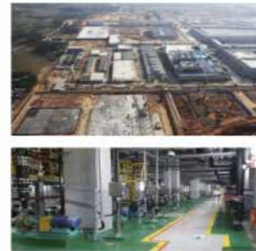
Name: SEVT Metal3D Glass Project Location: Thai Nguyen, Vietnam
