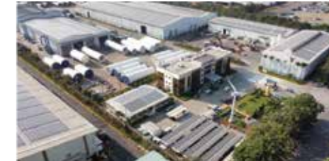
Name: CS Wind Factory Location: Ba Ria – Vung Tau Province, Vietnam
